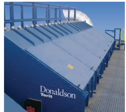
CPC - Grain Tripper Conveyor 18,700 cfm (31,765 m 3 /h)
