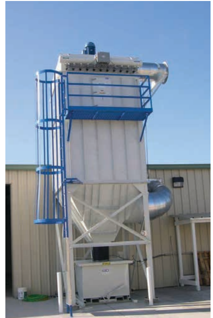
FS on Woodworking 20,000 cfm (33,973 m 3 /h)
