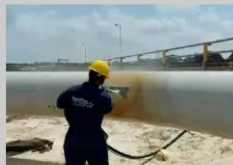
Running/Charged Pipeline Surface Preparation
