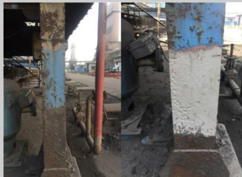
Before and after application of Vapor Abrasive Blasting
